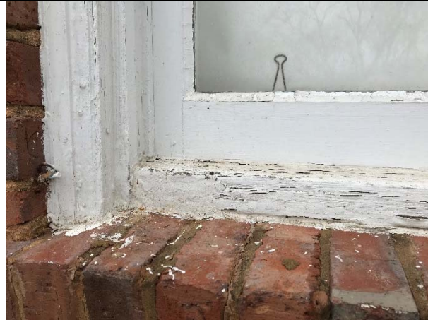
2. Typical rotted and damaged wood windows throughout the Jail.
