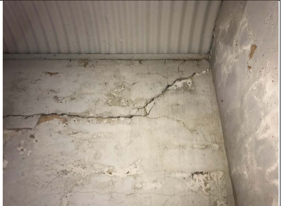
6. The exterior crack in picture #4 is starting to extend through the brick mass wall to the inside.
