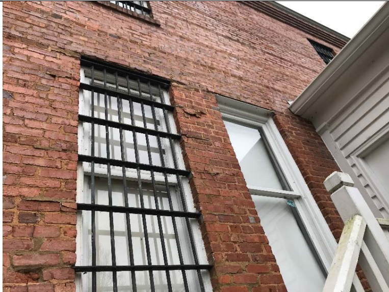
3. Steel security bars that are spalling the face of the brick off at the connection points.
