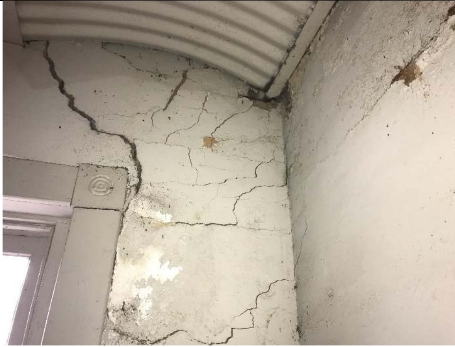
5. The exterior crack in picture #4 is starting to extend through the brick mass wall to the inside.
