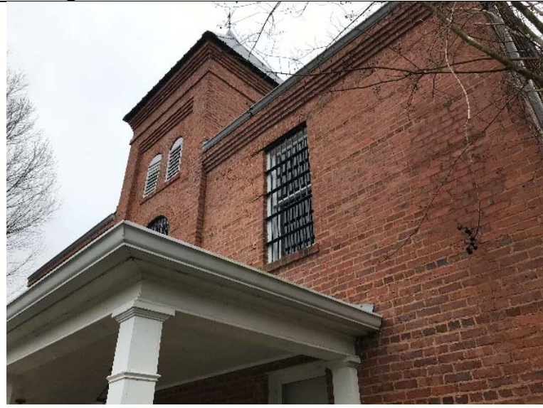
4. Steel security bars that are spalling the face of the brick off at the connection points. And large crack at corner.
